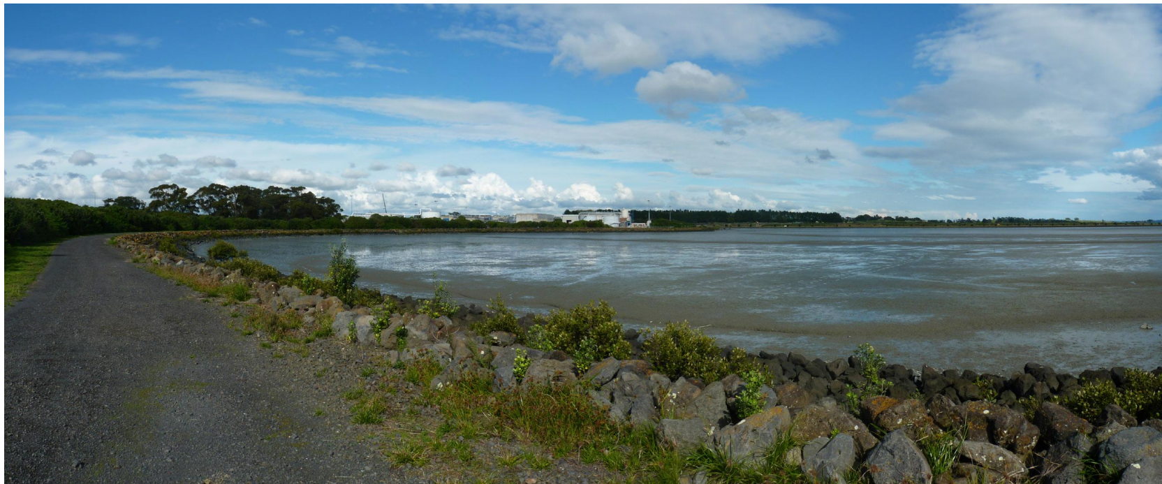
View of WWTP & Coastal Walkway
