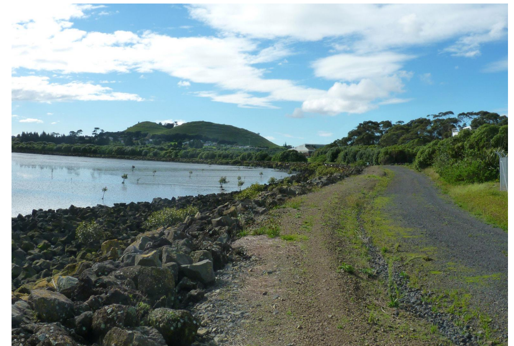
View of Proposed Emergency Pressure Relief Site
