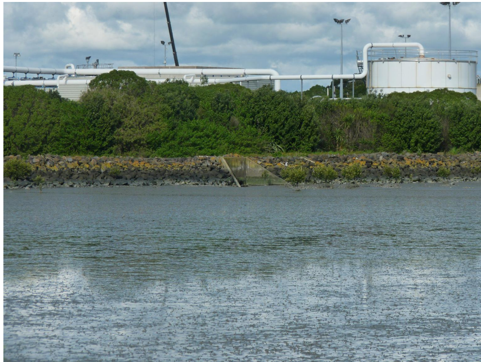
View of existing outlet & WWTP from Coastal Walkway
