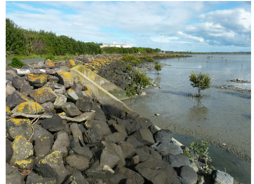
Existing outlet structure intergrated with rock rip-rap sea wall
